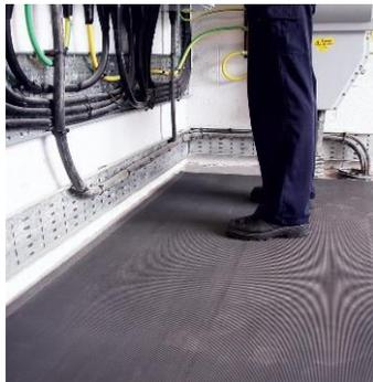
These items are a rubber floor covering or mat that offers protection and insulation in any given area you may find yourself standing in that puts you at a risk of running electrical hazard conditions. These mats are made with blended materials that are dielectric, meaning that the material has much higher internal resistance and integrity to withstand higher voltage output. These should be tested after approximately every 2 years.
